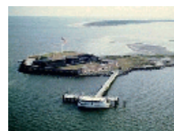
Fort Sumter National Monument Charleston, South Carolina
